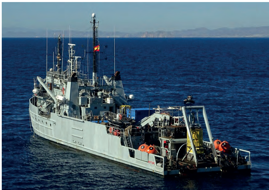
Despite its age, the Neptune A-20 continues to accomplish the missions it was designed for.
